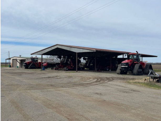
Large equipment shed
