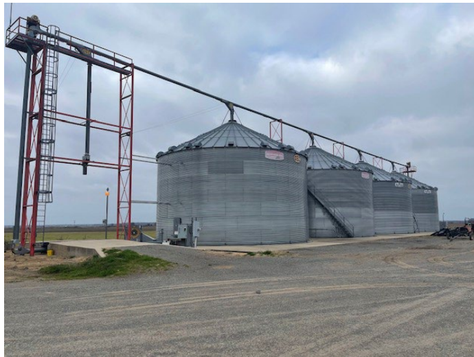
Large grain storage complex with loop system
